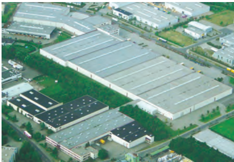
Logistic Center (approx. 60.000 m 2 )
